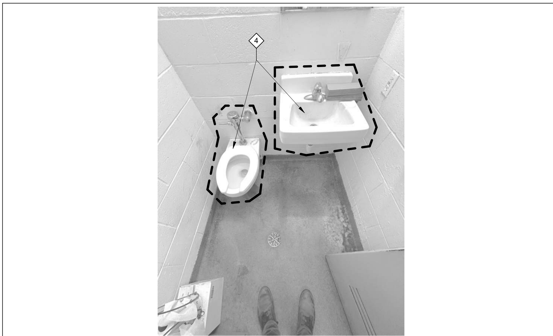
OFFICER RESTROOM - DEMO PHOTO #8 | R16
